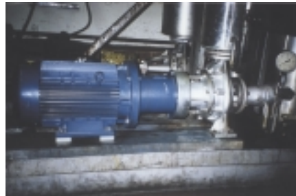
ZTK pumps with magnetic couplings for pumping heat transfer oil.
