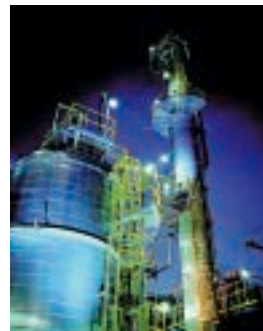
Process and Chemical
